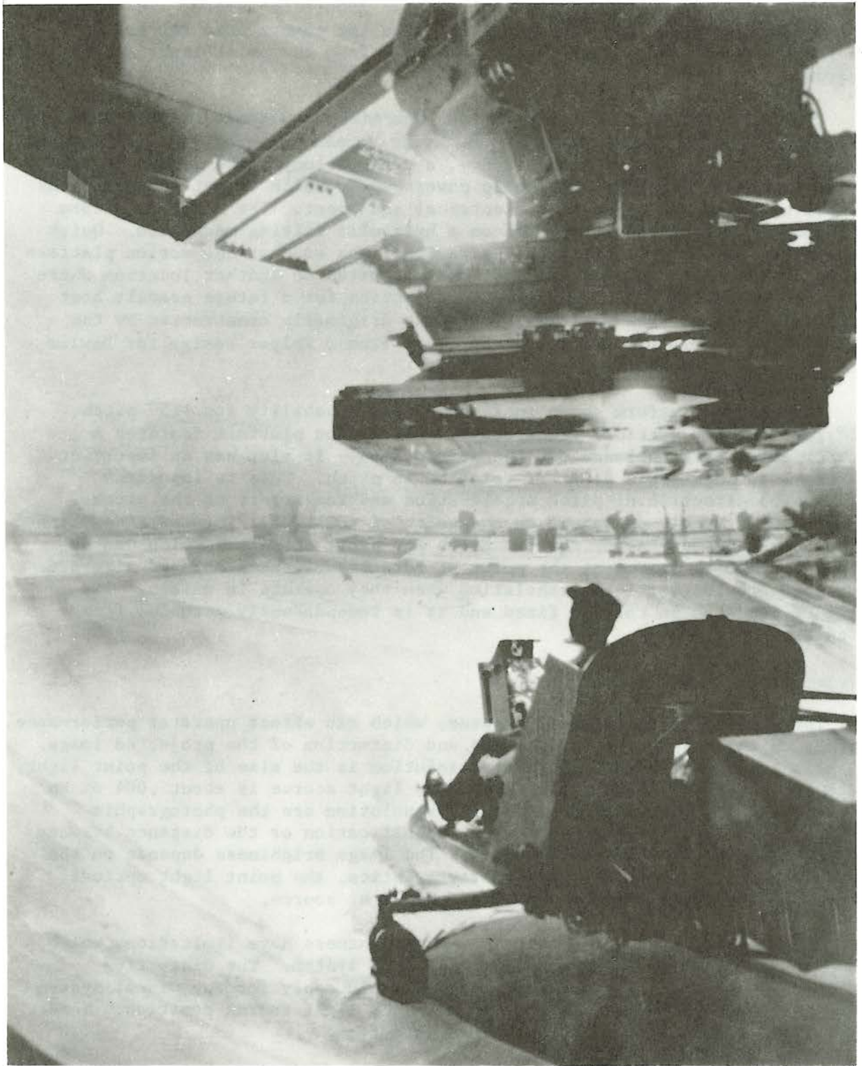
Figure 6. NAVTRADEVCCEN Devide 2-FH-2 Point Light Source Helicopter Trainer
