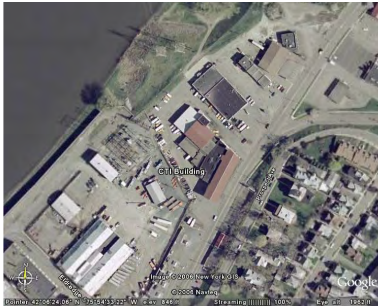
Figure II-1 CT&I Site From Above
